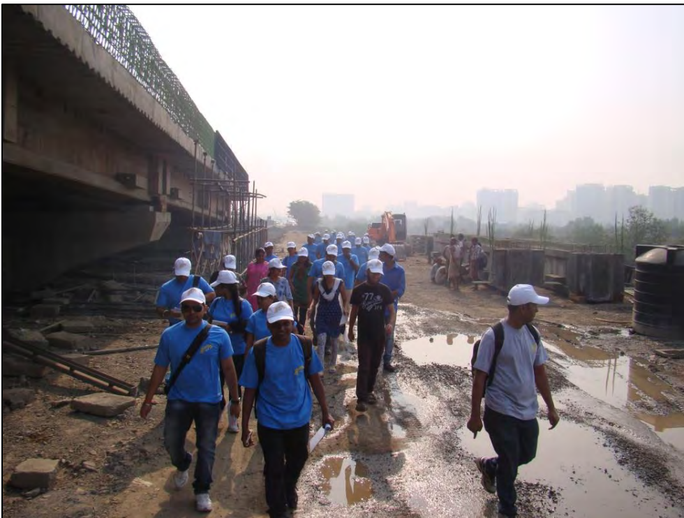
Picture No. 10: Construction activity just besides the mangrove habitat
