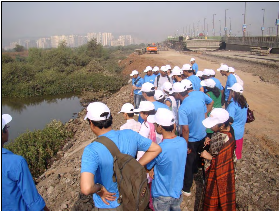
Picture No. 9: Dumping of debris at mangrove patch.
