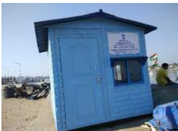
FRP cabin for security guards
