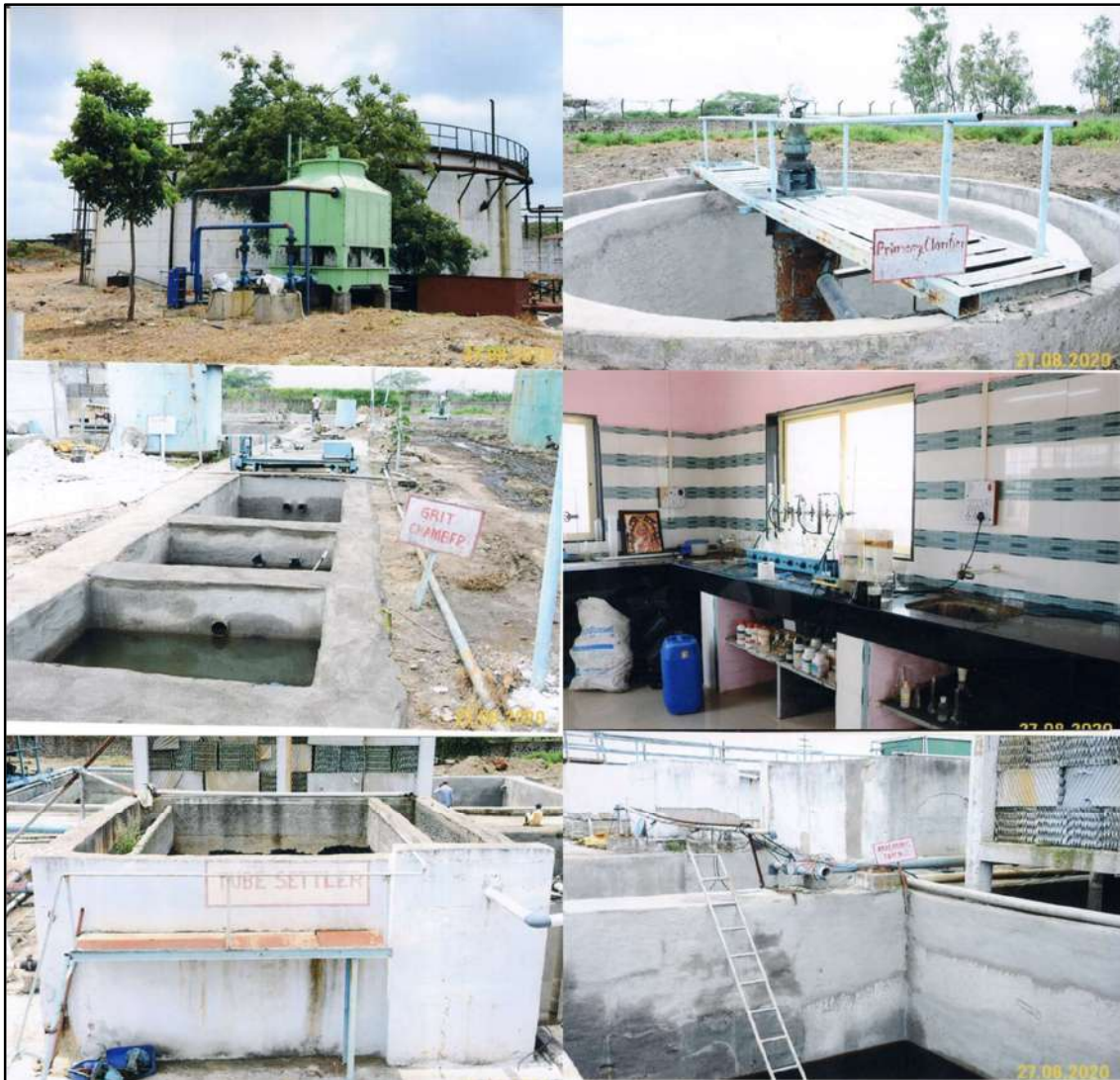
Figure 3 Photos of Existing ETP
