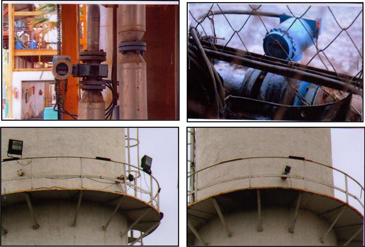
Figure 2.16 Online Continuous Monitoring System
