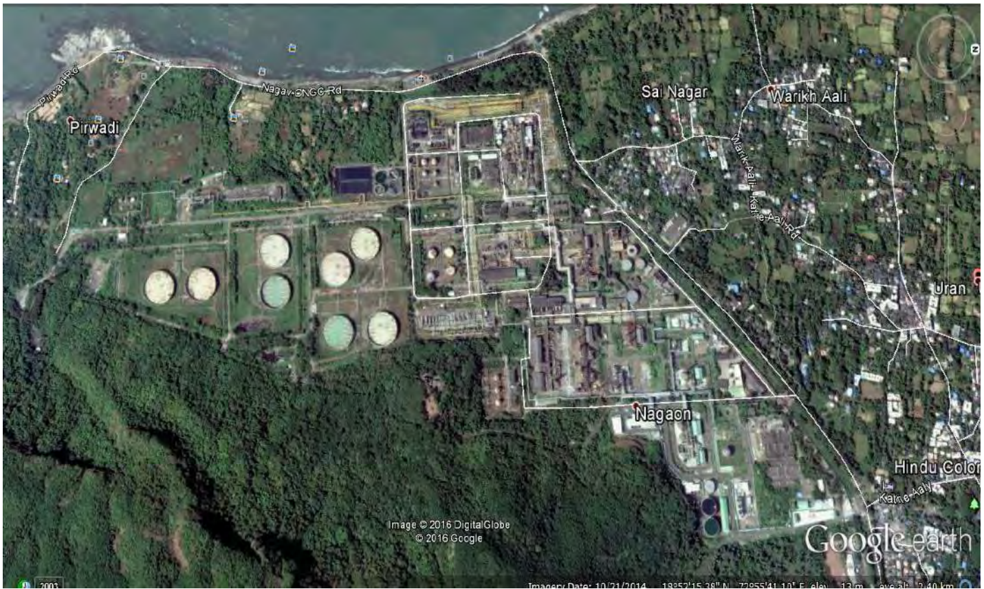
Fig. 1.1: Google Earth Image of the Existing ONGC-Uran Plant
