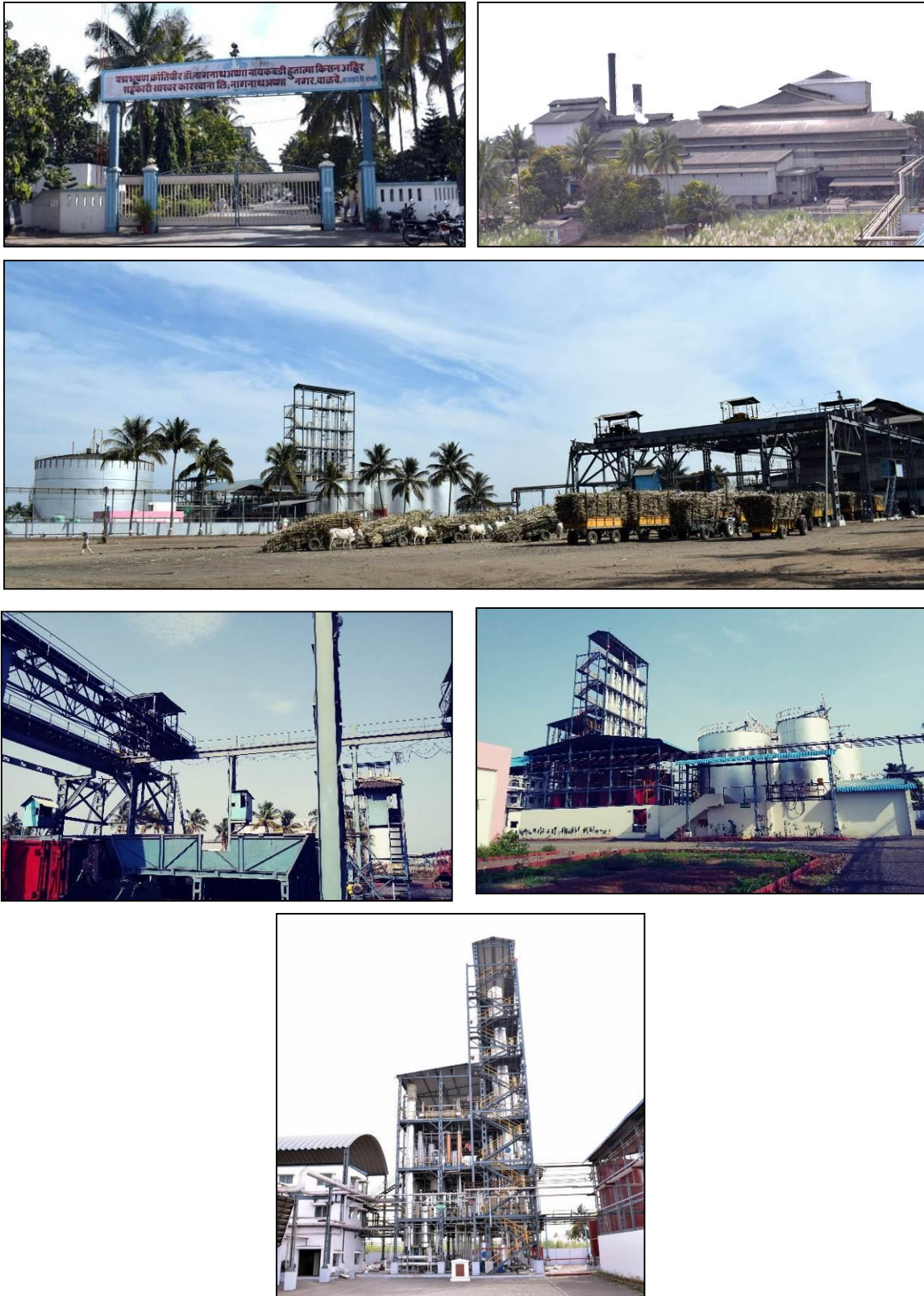
Figure 4: Existing factory photographs
