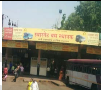
Swargate Depot (Kerbside)
