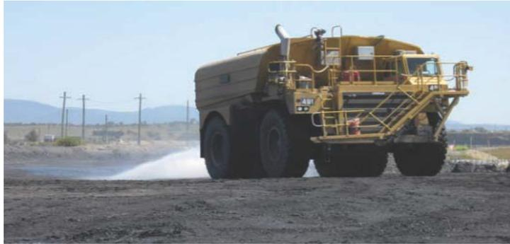
**Figure 1 : Road side sprinkling of dust control agents**
