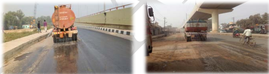
Application of Dust Suppressant using Tanker at Delhi
