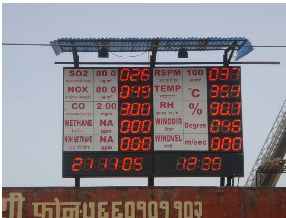
Display board of continuous air monitoring station at Vashi
