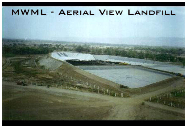
An aerial view of landfill site at MWML Talaja
