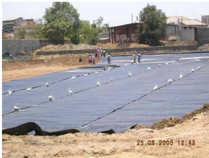
Secured Land-fill Work in Progress
