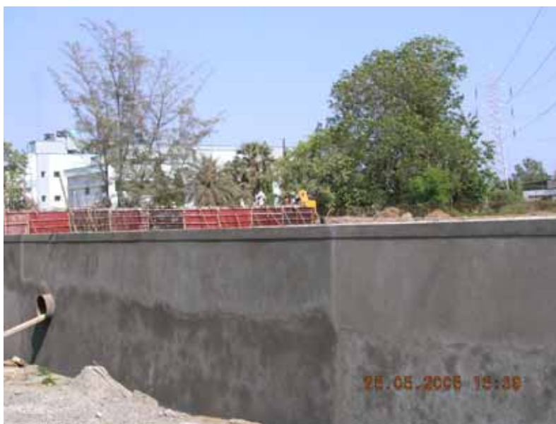
Construction of New 25 MLD CETP at Tarapur
