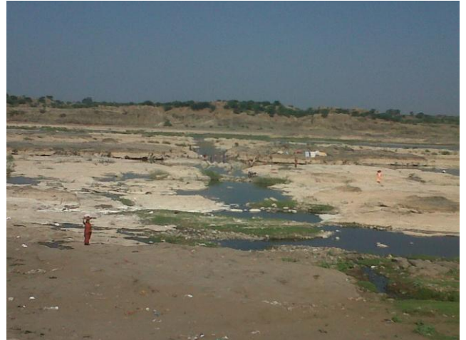
Tapi Near Railway Bridge Bhusawal
