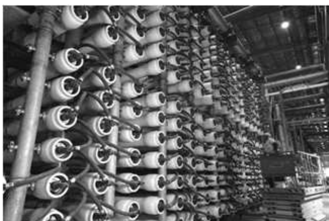
Figure 8 RO Plant showing stacking of RO membranes
