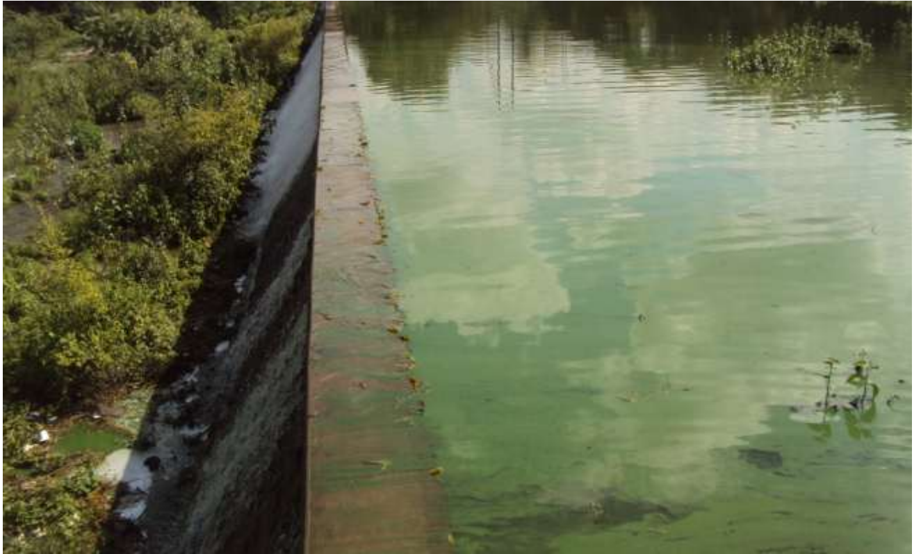
Figure no. 1.2 Overflow weir of Ambazari Lake
