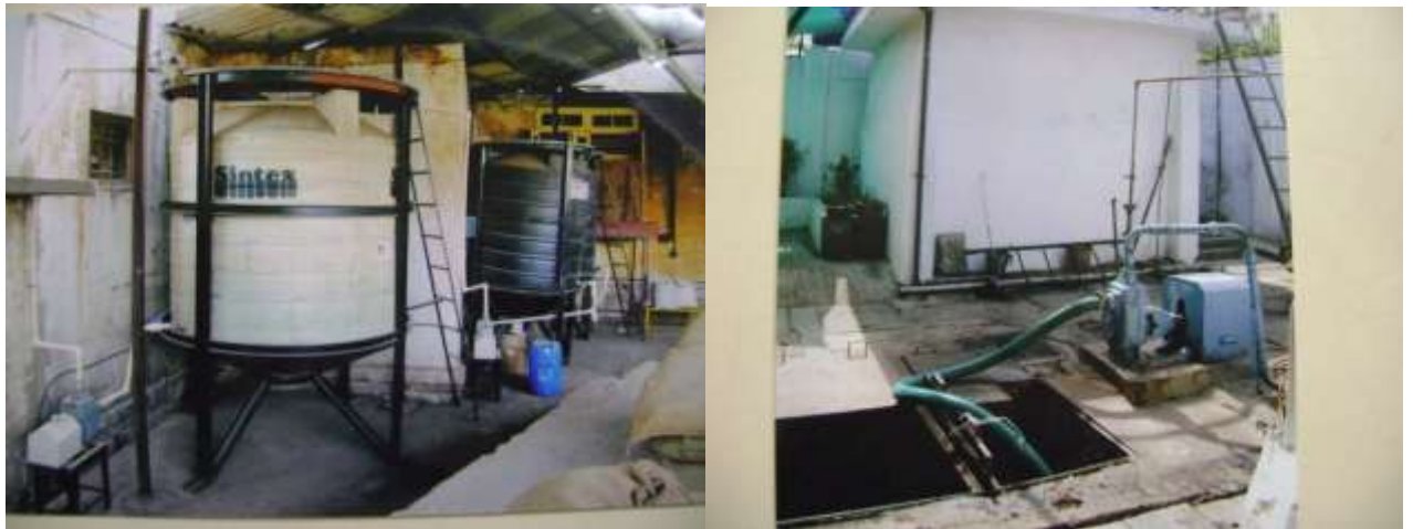
Figure no. 6.6 :- Wastewater Treatment Plant Installed at M/s. Shree Baidyanath Ayurved Bhavan Pvt. Ltd., Nagpur
