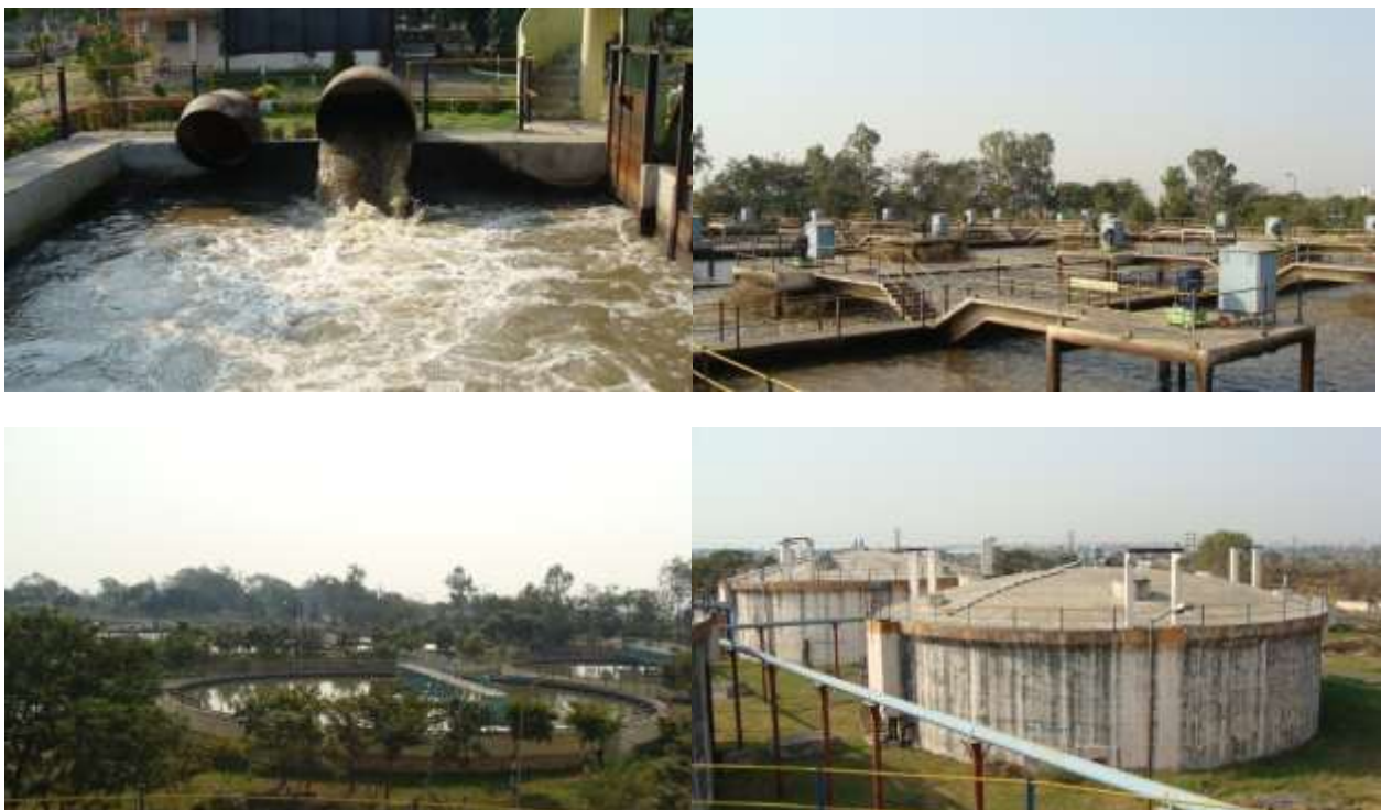
Figure 6.1 View of sewage treatment plant-Bhandewadi (100 MLD Capacity)
