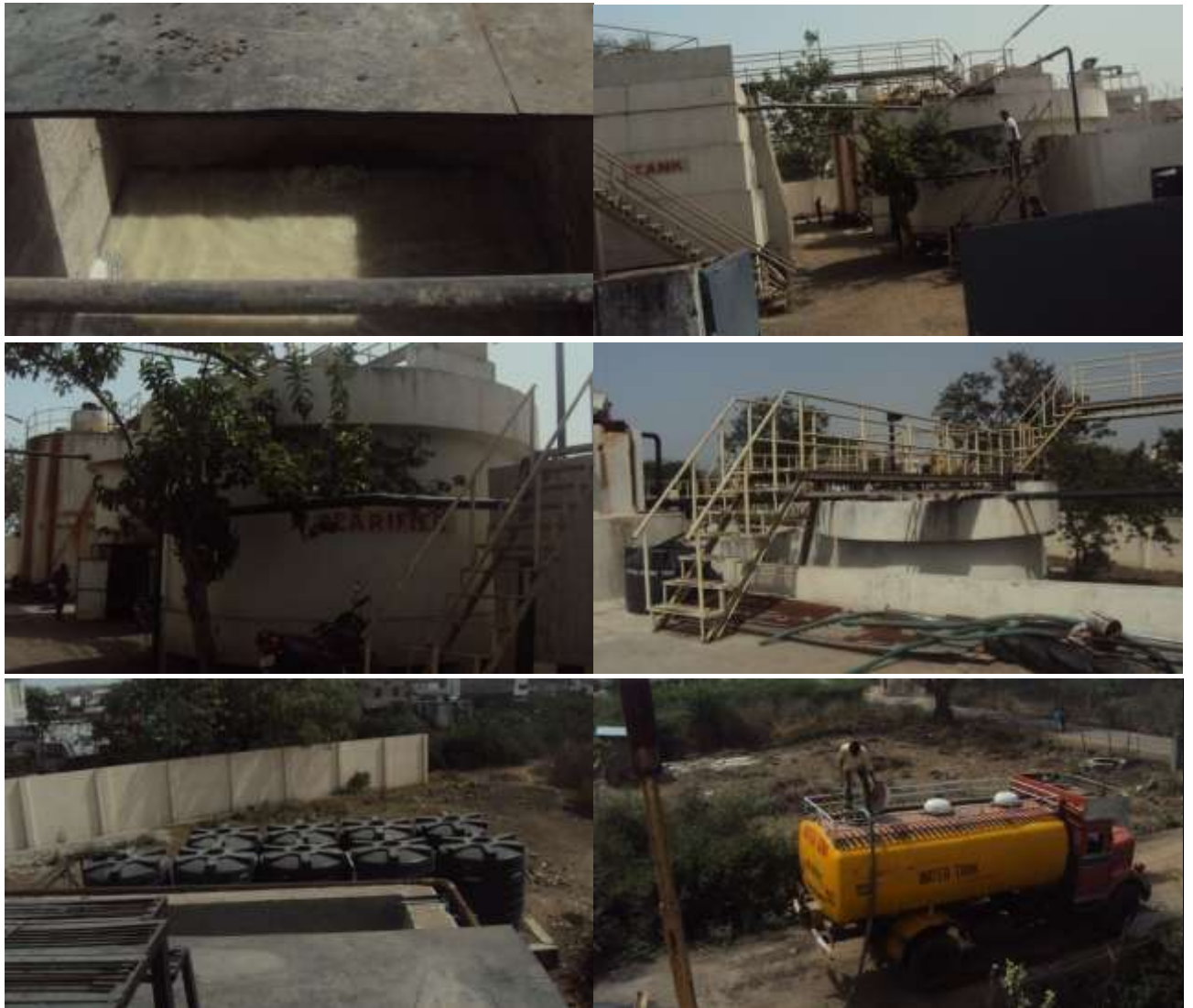
Figure no. 6.4 :- Wastewater Treatment Plant Installed at M/s. Dinshaw's Dairy Food Products Ltd., Gittikhadan
