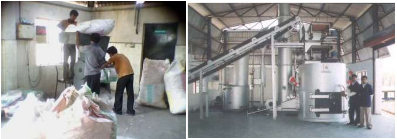
Figure no. 6.2 Biomedical Waste Plant (Shredder & Incinerator) CBMWTSDF
