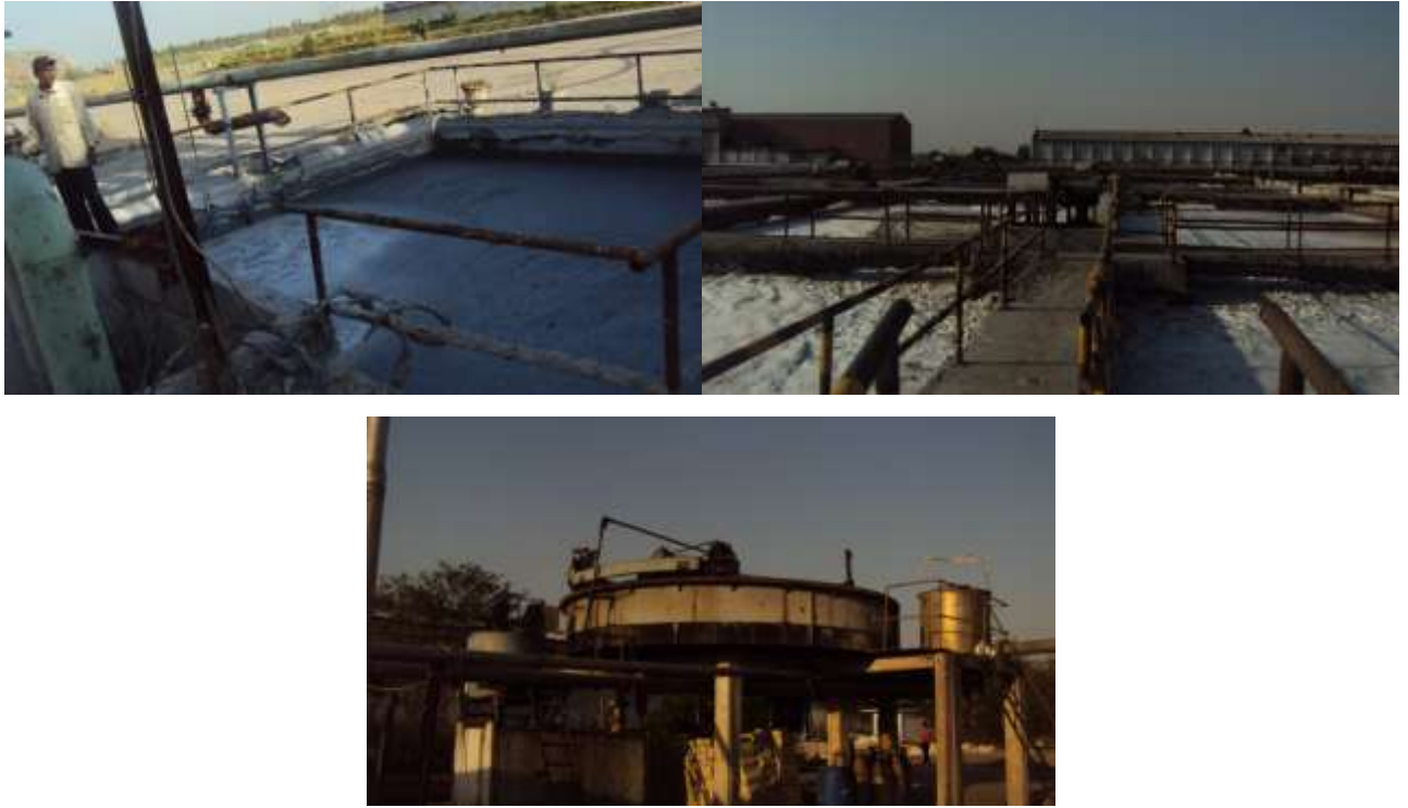
Figure no. 6.7 :- Wastewater Treatment Plant Installed at M/s. Murali Industries Ltd., Vadada, Tq. Kamptee
