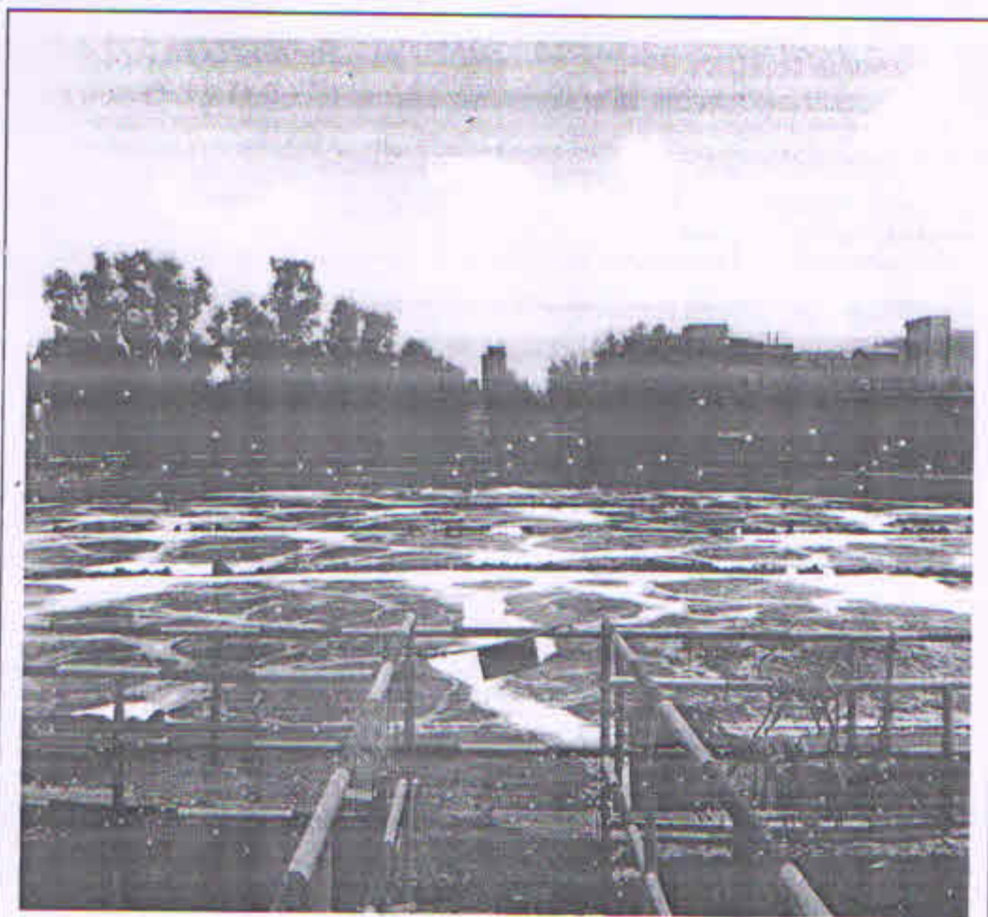
Figure 2Roha Industrial Association CETP
