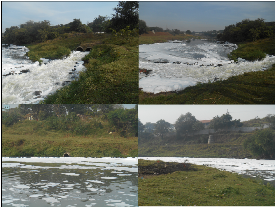
Photo 6: Extensive foam formation at the discharge of Tapovan STP in Godavari.
