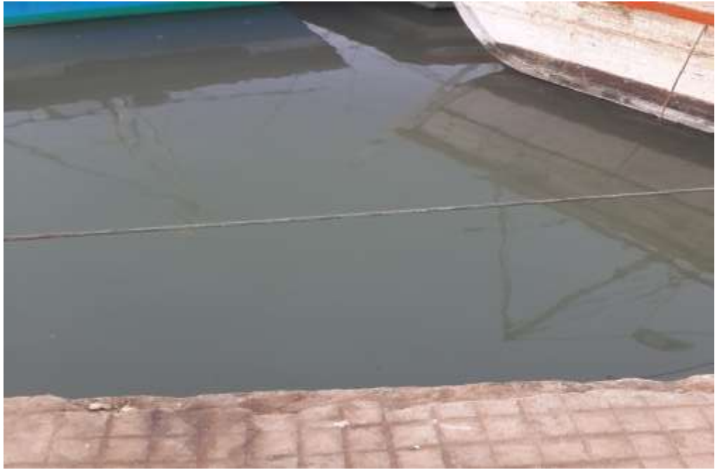
Figure 3.18.1: Fishery Harbour at Mirya Bay, Ratnagiri
