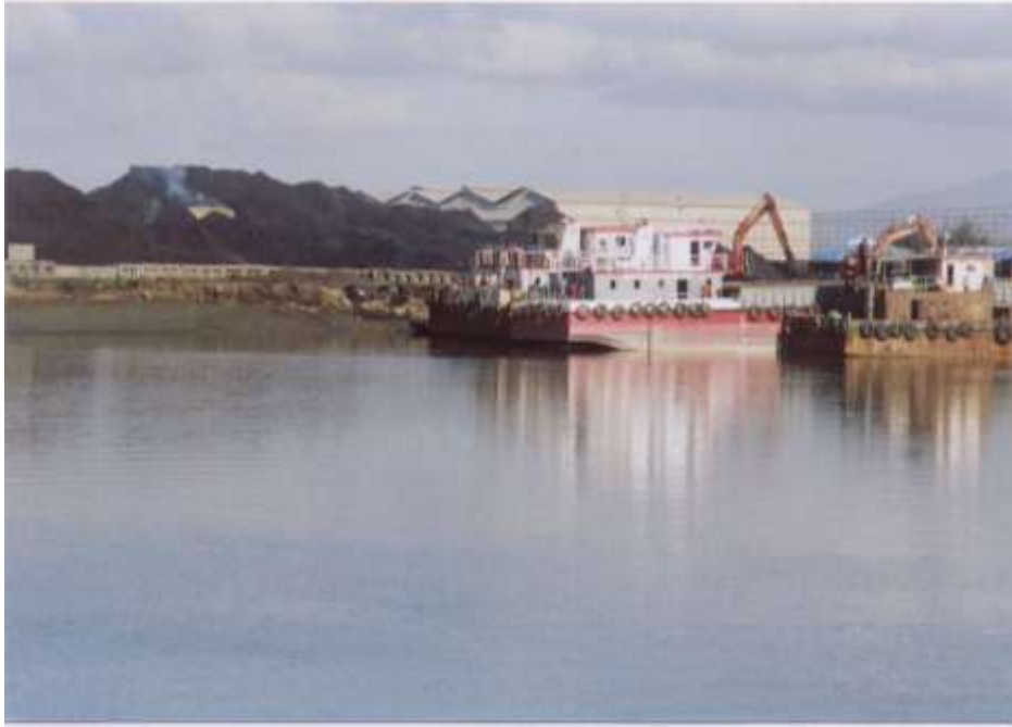
Figure 3.11.2: The PMP Port located at Dharamtar in Amba Estuary
