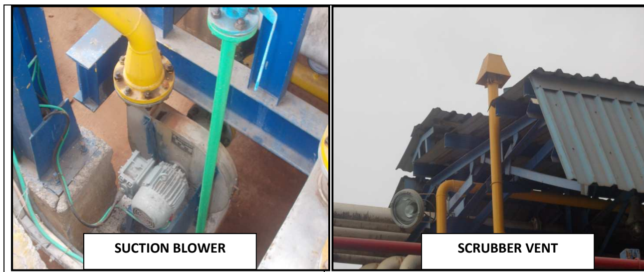
Figure 4.2 Photographs of Vent Collection & Scrubber System Provided
