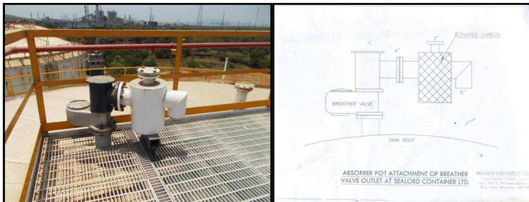
Figure 4.1 Breather Valve on VFR Tank with Activated Carbon Pot
