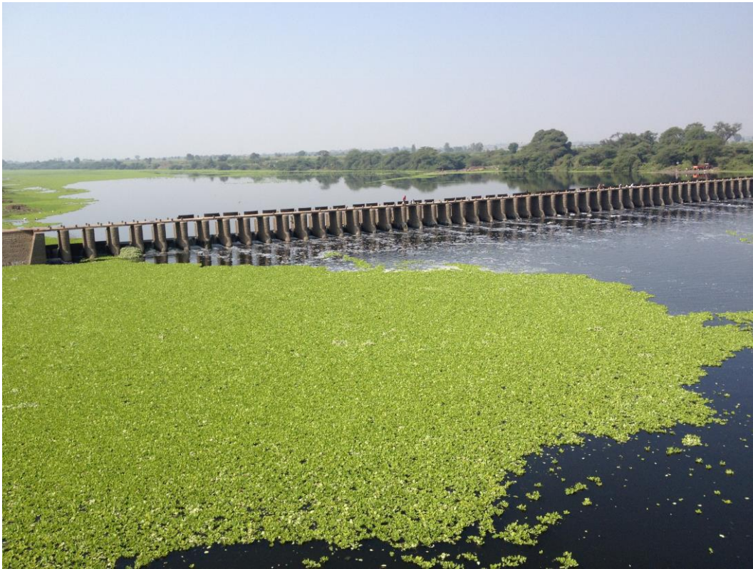
Bhima river under Kedgaon – Ranjangaon bridge
