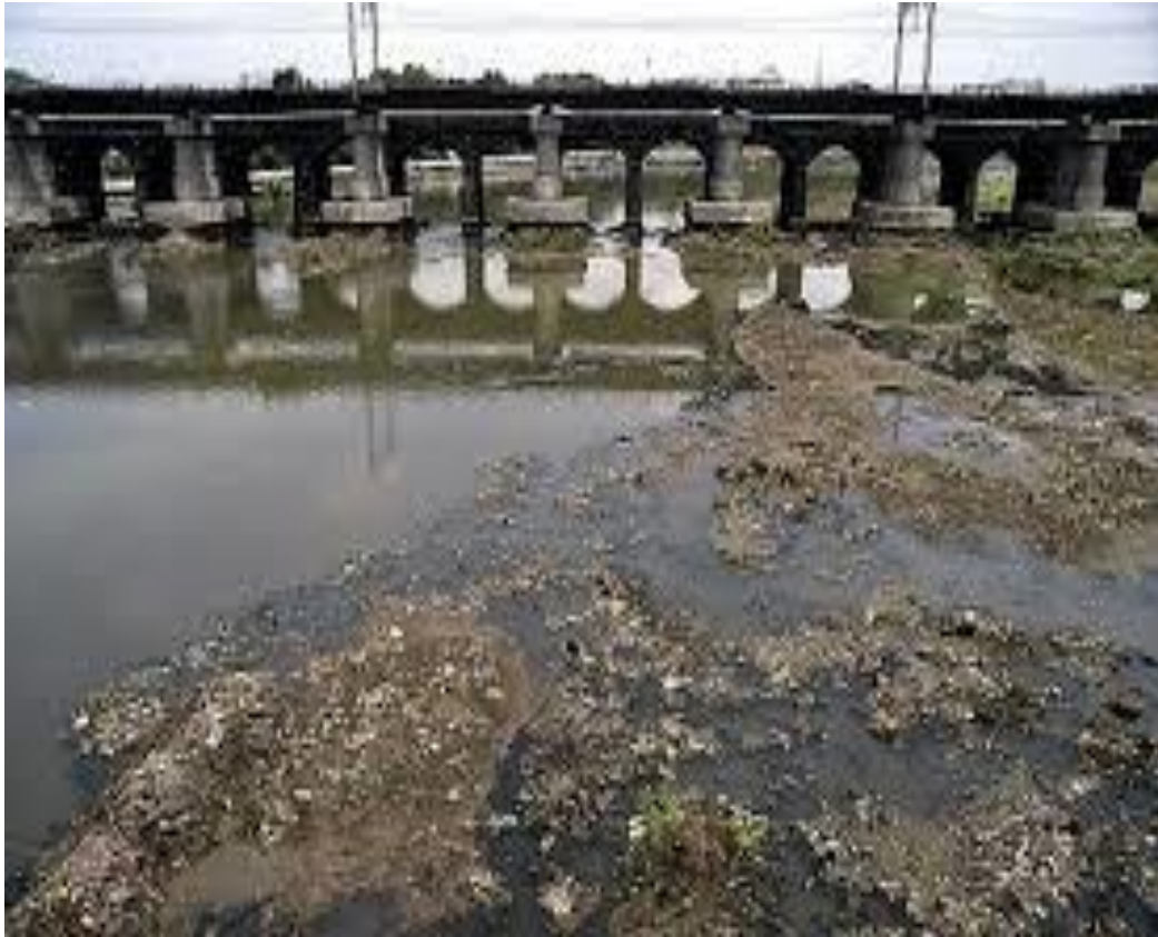
Mutha under Sangam bridge
