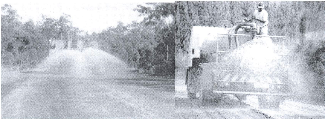
Figure 4: Application of dust suppressants for unpaved roads
