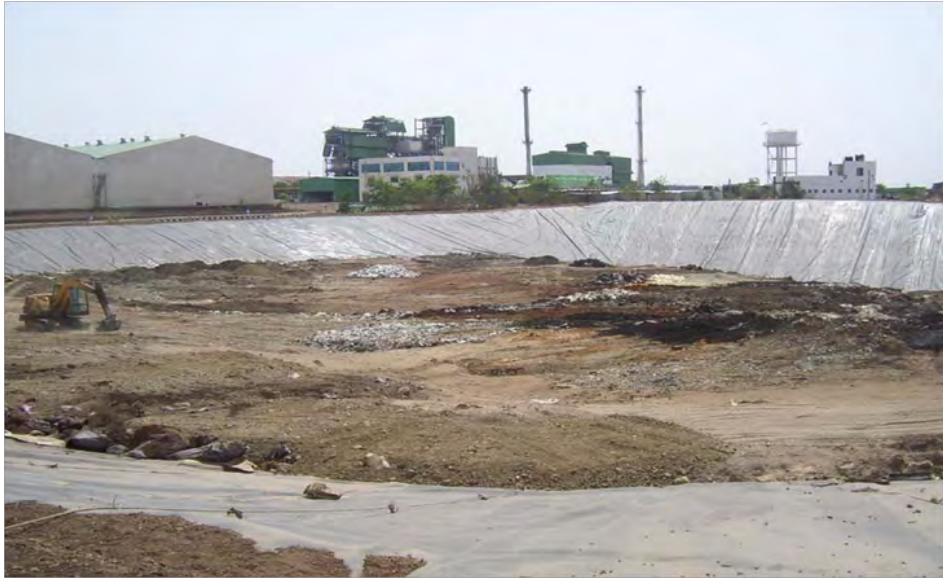
Picture III: Common HW Landfill site at M/s. Maharashtra Enviro Power Ltd, Ranjangaon Dist: Pune
