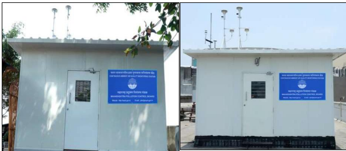
Fig. 5.1. Continuous Ambient Air Quality Monitoring Stations at Colaba (left) and Kurla (right) in Mumbai.
