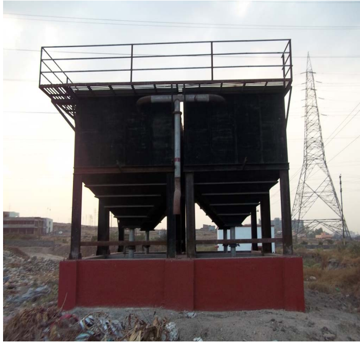
Leachate Collection system
