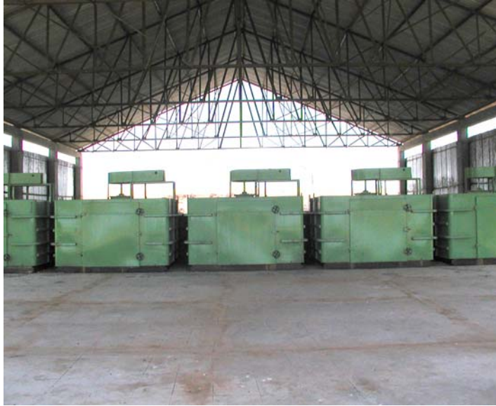
INSTALLATION OF VESSEL
