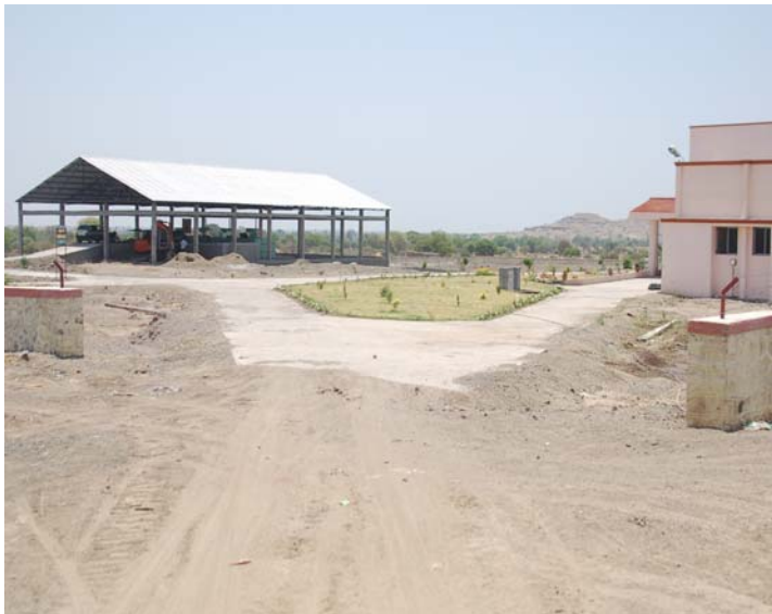
INTERNAL ROAD AND OVERVIEW OF SITE
