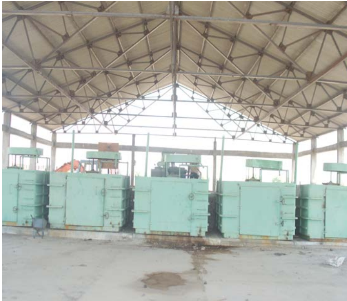
INSTALLATION OF VESSELS
